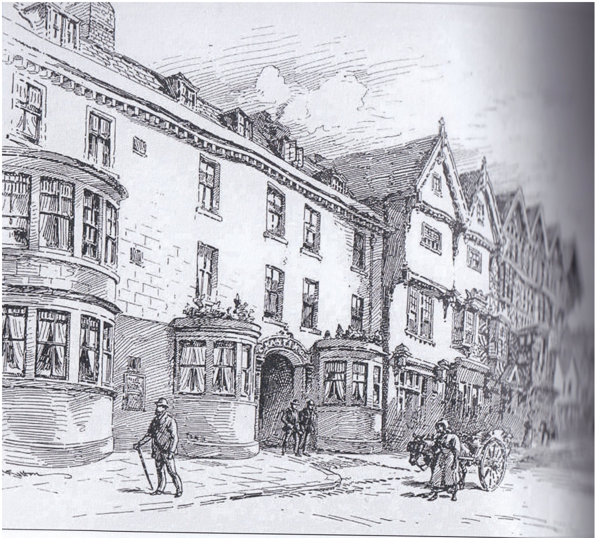
The Swan, Shaw's House and High House (by F.G. Sutton).
